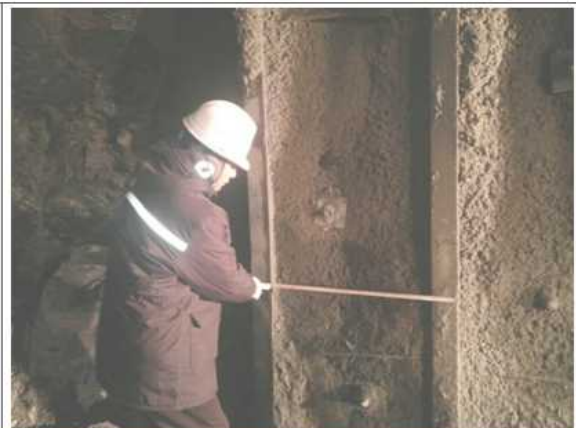
Rock Bolt, Shotcrete 상태점검
